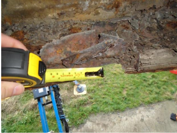
Condition of span 2 lattice structure renders repairs unfeasible
